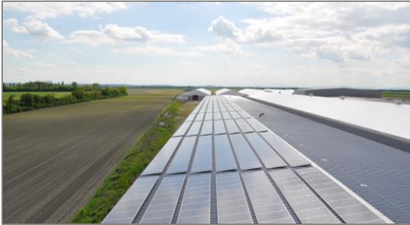
400 kW smart system in Vienna, Austria, powered by Tigo Energy.
